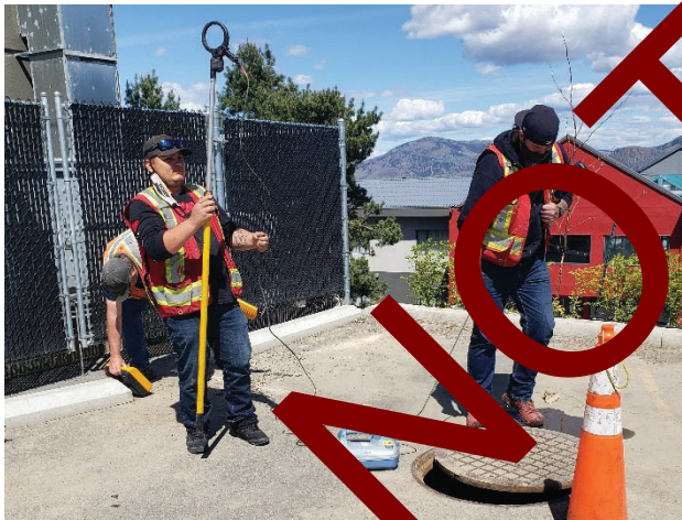
Using a Clamp Extension Rod to reach a target cable
