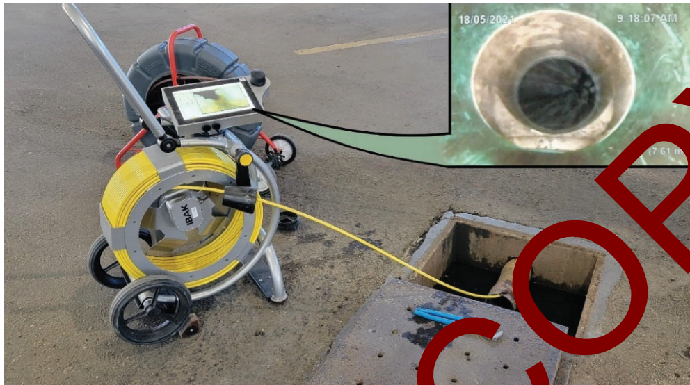
A camera sonde inside a drainage line
