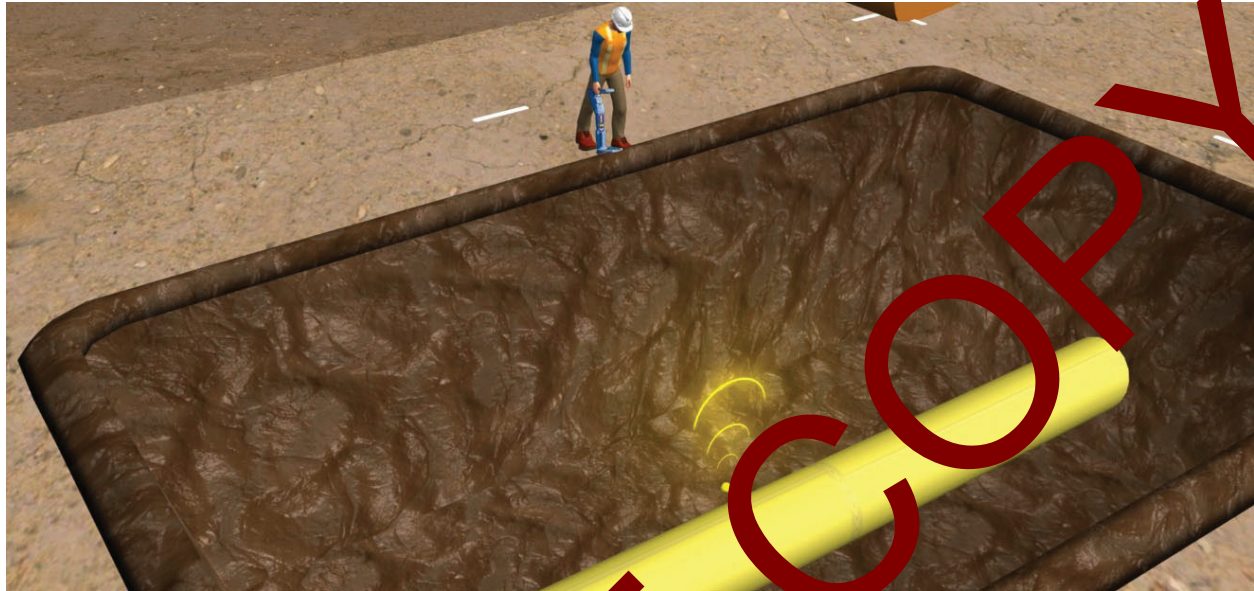
Marker ball placed at pipe weld
