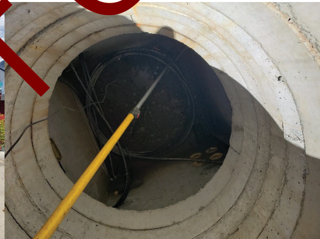
Using a Clamp Extension Rod to reach a target cable
