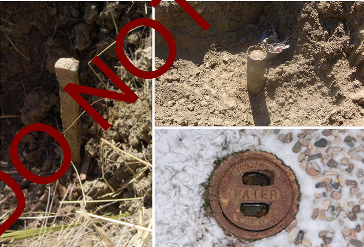
Survey pin (left); well casing (top right); water valve (bottom right)
