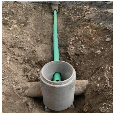
Catch basin tying into a main line manhole
