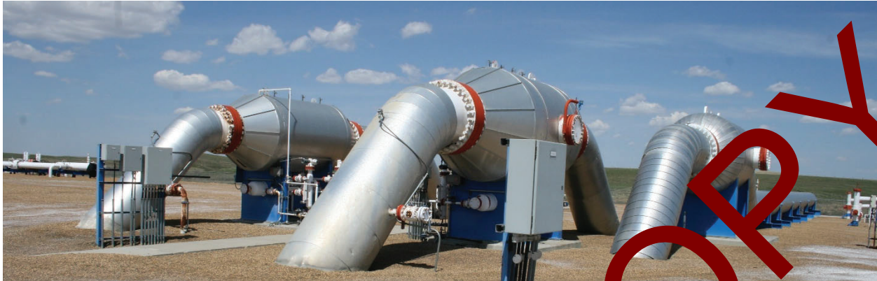
Pipeline risers within a compressor station
