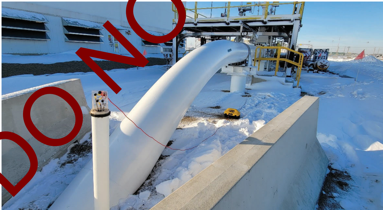
Using a high frequency on a cathodic test lead attached to a large diameter pipe
