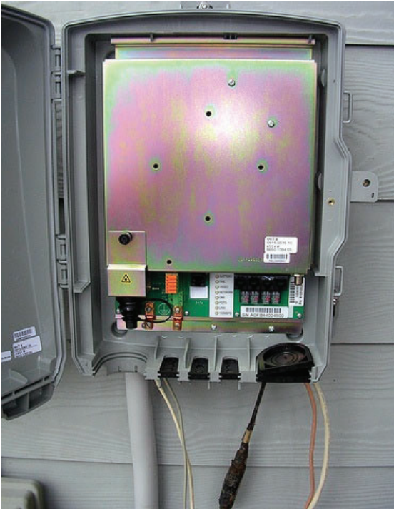
Customer optical network terminal (ONT)
