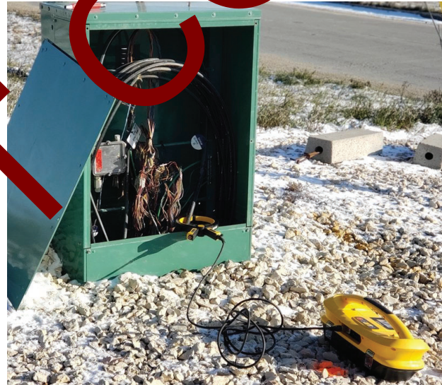
Inductive clamp around a fibre-optics cable
