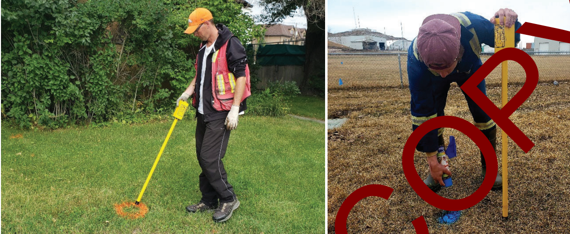
Using a magnetic locator (pin finder) to locate a water curbstop valve
